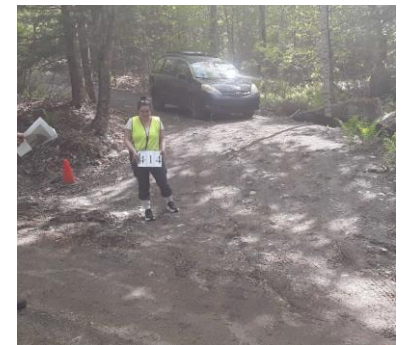
A high impact driveway site that is eroding into a stream to Threemile Pond
